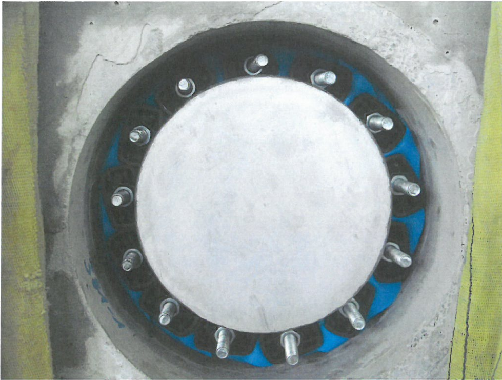
Figure 3: The link chain seal installed for sealing the annular gap
